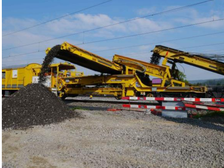
Figure 46. UMH placing excavated material
