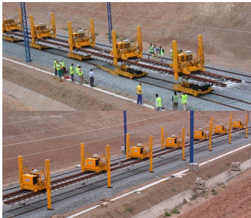
Figure 4. Set of gantries with motor bogies
