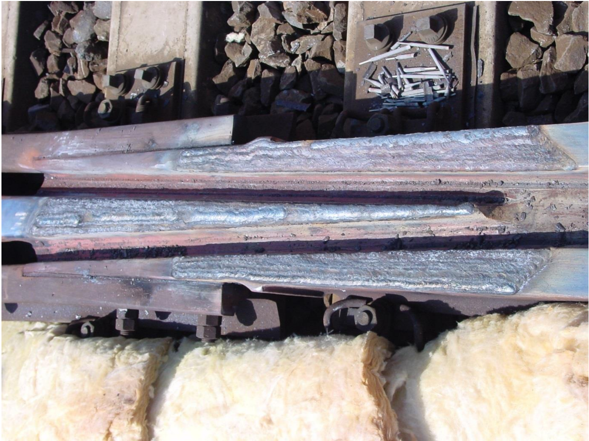
Figure 32: Welded-on overlay on the running surfaces of the frog [17]
