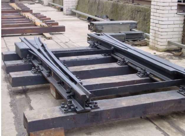
Figuur 2.14 Terugklapwissel ("Single-blade tramway switches,")
