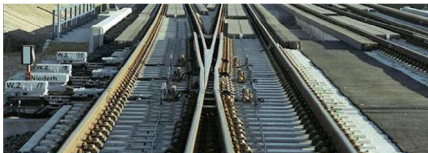
Figuur 2.5 Wissel in hogesnelheidsspoor (AgicoGroup)
